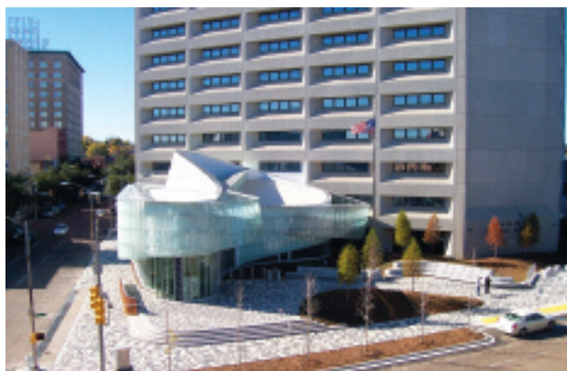
IBEW Local 480 members worked on the Dr. A.H. McCoy Federal Building modernization project in Jackson, MS.
